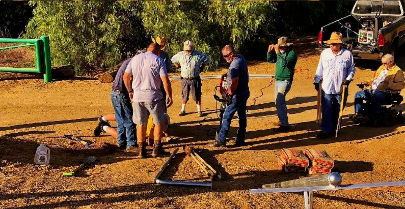
Gate-building work party– photos by Steve Gebler
