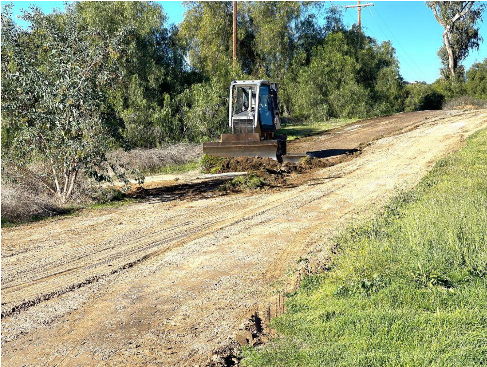
Jan. 8, 2024 saw our road graded and the gullies created by the rain erased. Thanks muchly! Photo courtesy Steve Gebler.
