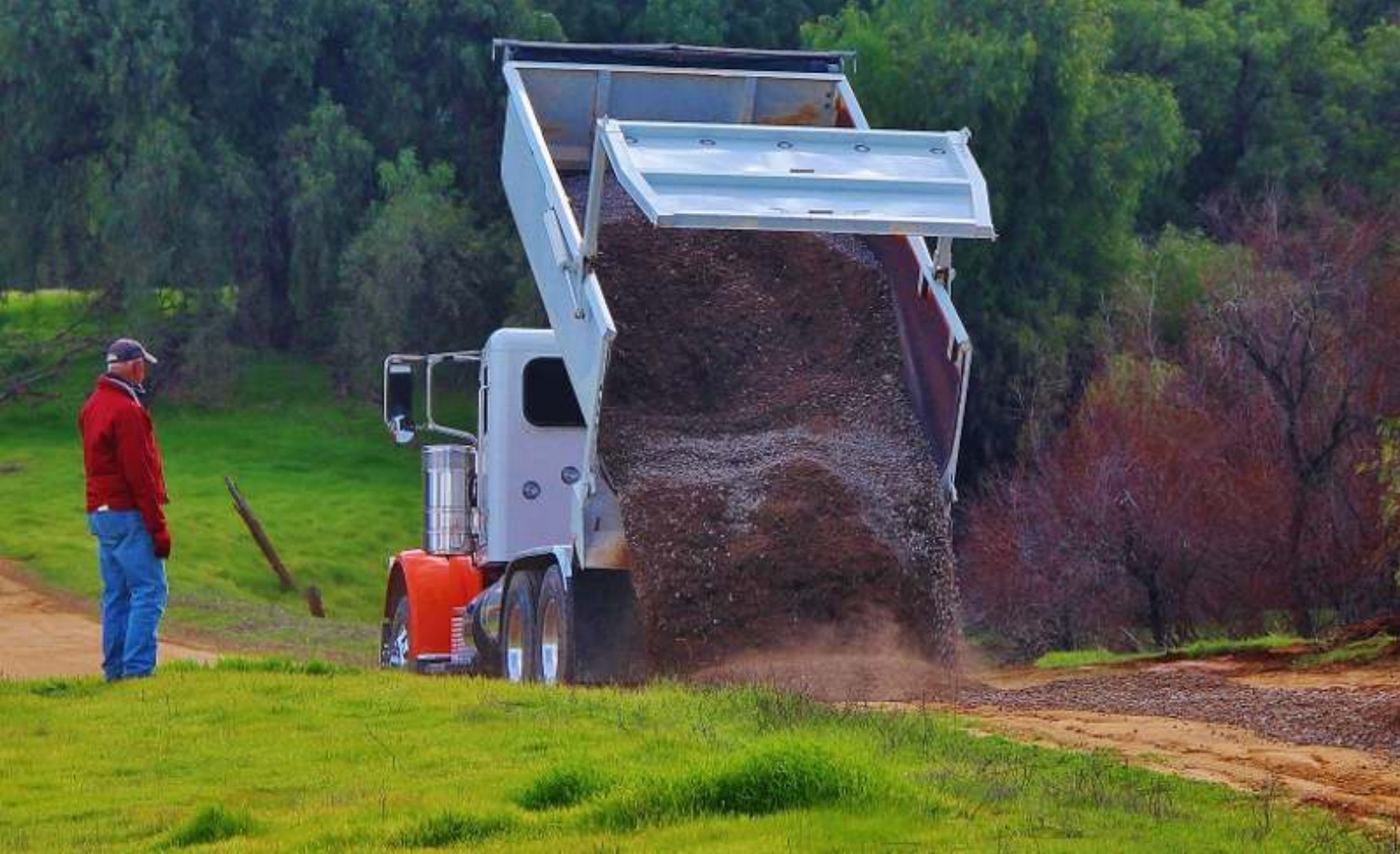
Some of the 150 tons of gravel applied to our road.
