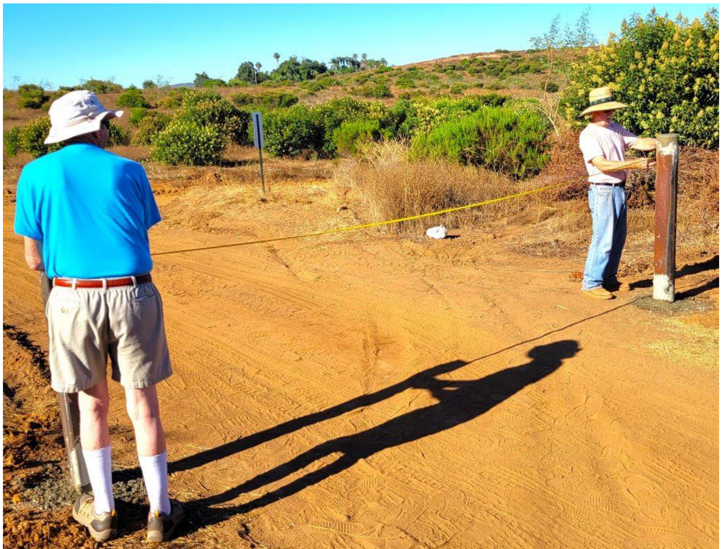
President emeritus Joe Villarreal setting the gate posts which are placed in concrete @ our Valley Center site.
