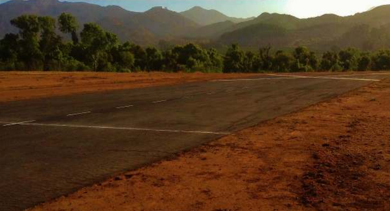
Our runway was resurfaced and painted on June 11 + 12, 2018. The next 8 photos were taken by David Drowns before and after its restoration.
