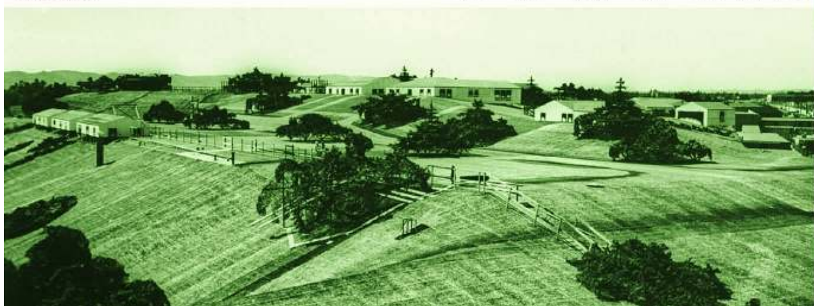
Here are concealed factories and assembly plants that may have been targets during WWII, including Douglas Aircraft. In a short period of time the entire area of the factory was camouflaged. The Lockheed-Vega aircraft plant in Burbank was fully hidden beneath a complete suburb replete with rubber automobiles and peaceful rural neighborhood scenes painted on canvas. (Greg Wilson contributed this photo. He was just 23 when he took it in 1944. Happy 100th this year!) You don't look a day over 99!)
