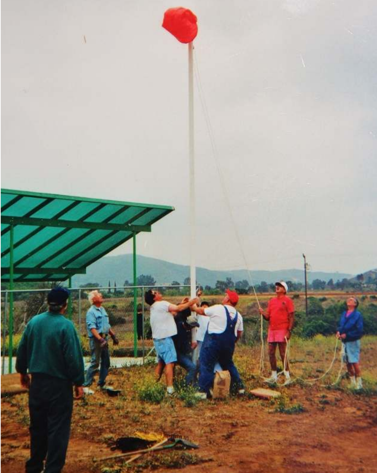
Bob and company raising the windsock pole-
