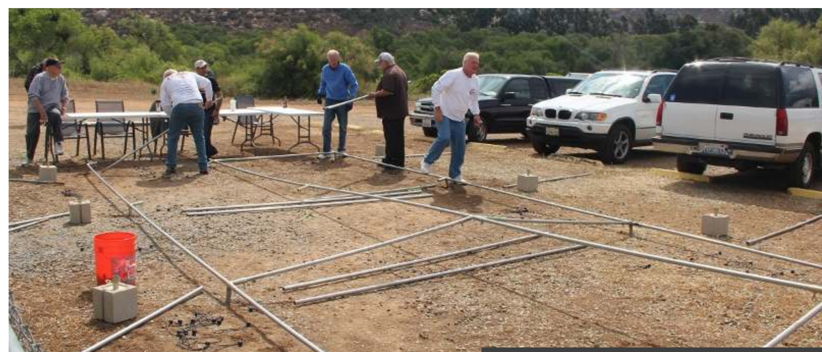
On May 22, the crew put up the “Big Top” for shade.
